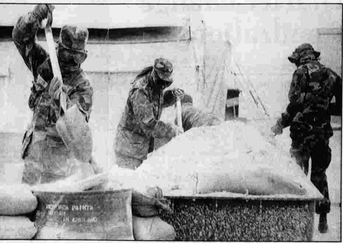
STIFFENING THE DEFENSES — Staff Sgt. Michael Martans, a member of the 103rd Tactical Air Command, fills oil drums with sand to form hardened bunkers on the flight line at "Carnel Lot," the largest air base in Saudi Arabia.
